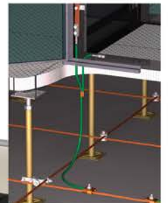
B Signal Reference Grid (SRG)
